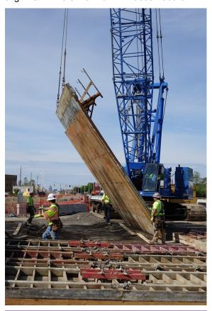
Construction workers adjust concrete forms to set the Gratiot Avenue bridge abutment walls. The pattern for the Constellation aesthetic finish is part of the form and will be imprinted on the new walls.
