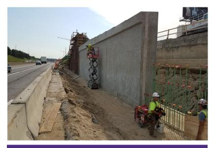
The new south abutment wall of the Chene Street bridge. The beams will sit atop the wall. Notice the wall's design? It's an aesthetic finish called Constellation that will make the bridge more attractive.
