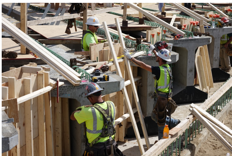
Formation of the diaphragm between the beams on the Gratiot Avenue bridge. The T-shaped structures are the ends of the concrete beams.
