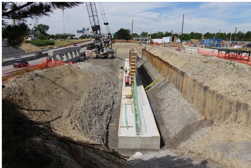
Installation of reinforcing steel and formwork for the Chene Street bridge abutment B north of I-94.
