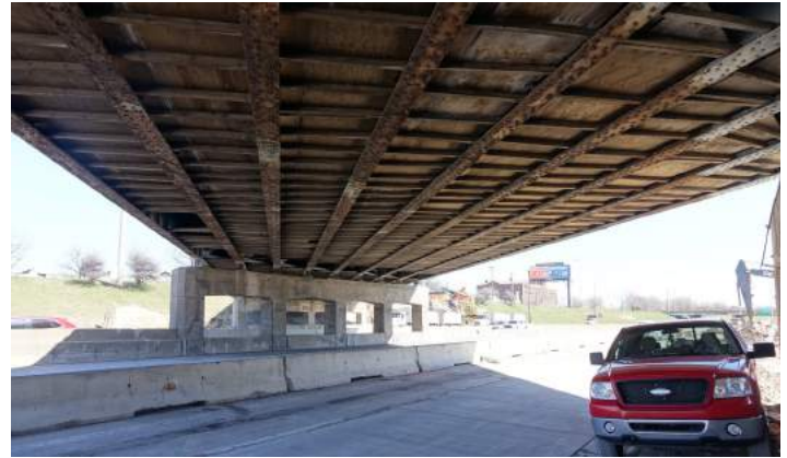
The old Gratiot Avenue bridge originally constructed in 1958.
