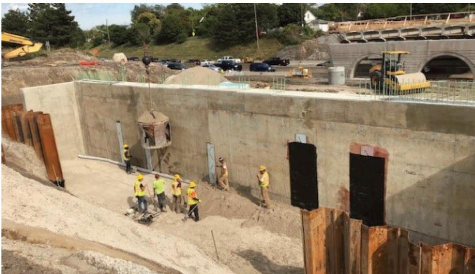
Members of the GLEG team inspect the Concord Street bridge when it was rebuilt in 2019. (Photo Description: A work site scene. Seven people in high-visibility vests and hardhats work around an abutment wall. The bridge has its support walls built but no span on top yet.)
